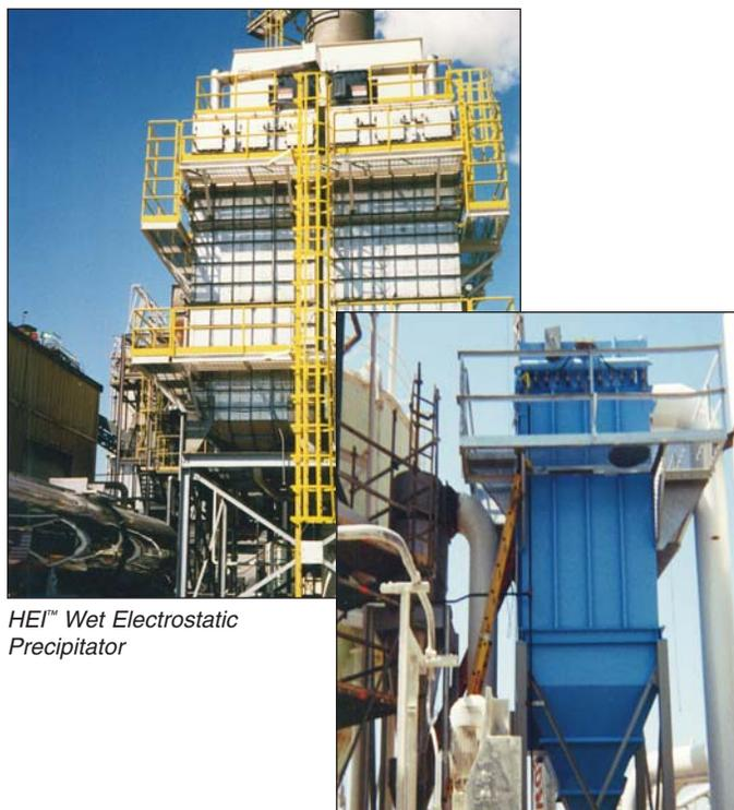
HEI™ Wet Electrostatic Precipitator
