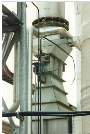
In operation, scrubbing liquid is introduced to the scrubber through fully open nonclog pipe headers. The contaminated gas enters through the top of the venturi scrubber with the scrubbing liquid in a cocurrent flow arrangement. The gas and scrubbing liquid then enter into a narrow throat section where a high-pressure drop accelerates the gas and shears the scrubbing
