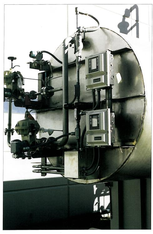
Industries for an alternative solution, the company proposed a system that eliminated multiple scrubbers and the hazards and cost of dangerous chemicals. It recommended using its ScrubPac™ BIONOxSOLVER™ system, which includes its two newly developed products: the DRI-NOx low temperature catalytic converter combined with the BIONOxSOLVER™ NOx wet scrubbing solution.
