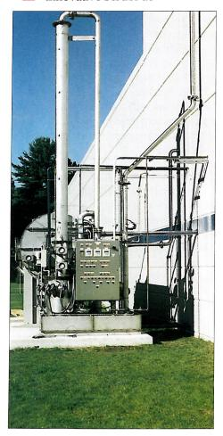
BIONOxSOLVER™ abatement system is enabling American Superconductor Corporation to treat the nitrogen oxide (NOx) emissions from a calcination process at its new, high temperature superconductor manufacturing facility (Devens, MA), in a cost-effective, environmentally responsible way.
