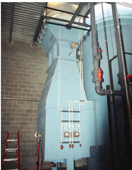
The Bionomic Industries Series 7000 venturi scrubber helps to eliminate odors at International Ingredient Corp.'s drying plant in Monroe, WI. Source: Bionomic Industries.
